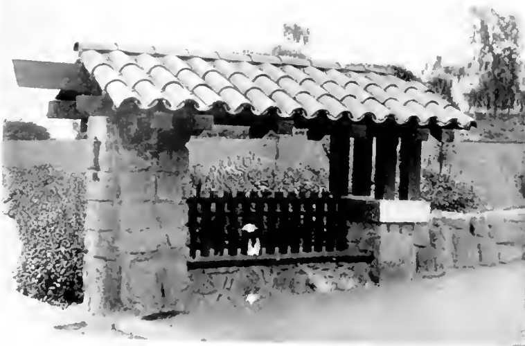
SEAT BESIDE A DRIVEWAY, WITH STONE PILLAR AND BASE AND A TILE ROOF.
