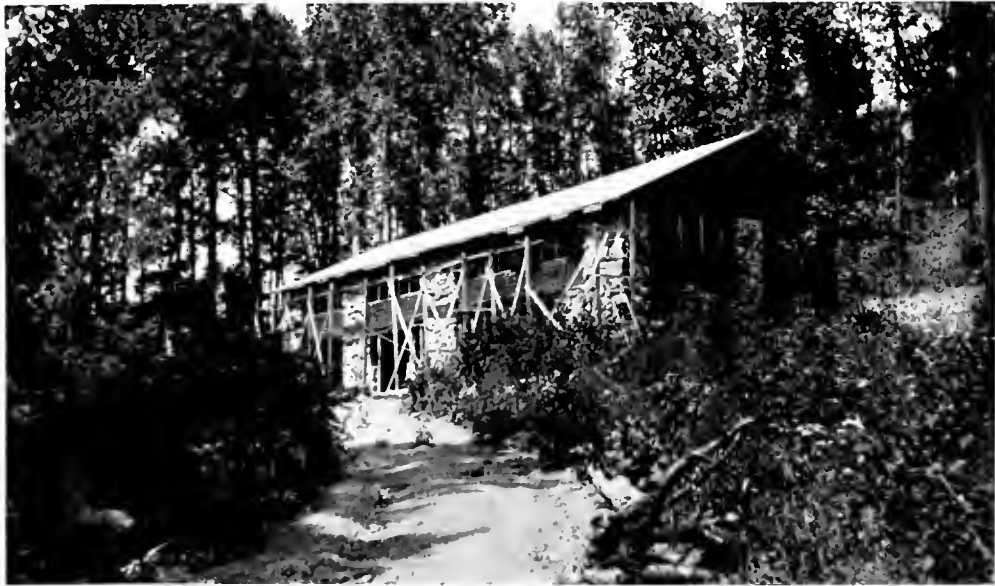
THE COW STABLE AT CRAFTSMAN FARMS, BUILT OF FIELD STONE: THE GROUNDS AROUND THIS STABLE ARE GRADED AND PLANNED, BUT AS YET UNPLANTED THE HORSE STABLE AT CRAFTSMAN FARMS IN PROCESS OF CONSTRUCTION: THE PLACING OF THIS STABLE IS ESPECIALLY INTERESTING ON THE SIDE HILL AGAINST THE WOODLAND BACKGROUND
