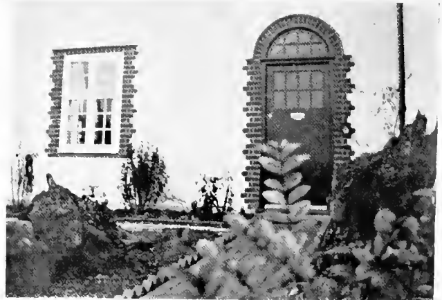
BRICK AND CON- CRETE HOUSE IN THE HAMPSTEAD GARDEN CITY NEAR LONDON. AN ES- PECIALLY INTER- ESTING COMBIN- ATION OF BRICK AND CONCRETE IS SHOWN IN THIS STRUCTURE. THE BRICK IS NOT ONLY USED FOR THE SUBSTANTIAL WALL AND FOUN- DATION, BUT AS A TRIMMING TO THE CONCRETE, FRAM- ING IN THE TWO LARGE BOW WIN- DOWS.
