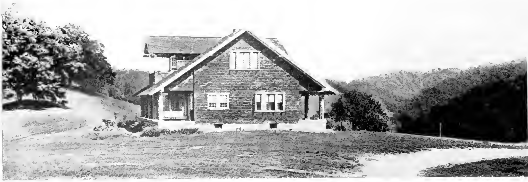
HOUSE OF MR. J. GORDON SMYTH, BUILT ON A HILLSIDE AT VAN LEAR, KENTUCKY.
