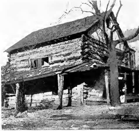
PI. II RESQUE CABIN IN JONCAIRE STREET. IT WAS ERECTED BY A FRENCH FARMER ABOUT THE MIDDLE OF THE EIGHTEENTH CENTURY.
