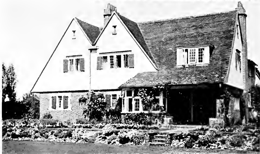
THE FRONT VIEW OF A CHARMING HOUSE IN THE GARDEN CITY AT LETCHWORTH, ENGLAND, IN WHICH BRICK AND CEMENT ARE COMBINED: IN THIS CASE THE BRICK IS NOT USED IN THE DEFINITELY ORNAMENTAL WAY, BUT AS A BASIS FOR THE FOUNDATION. THE FIRST STORY, THE PATHS, THE ENTRANCE WAY, THE PORCH SUP- PORTS, AS WELL AS THE CHIMNEY.
