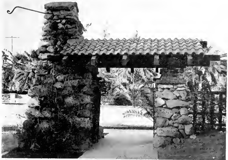
STONE GATEWAY WITH TILE ROOF.
