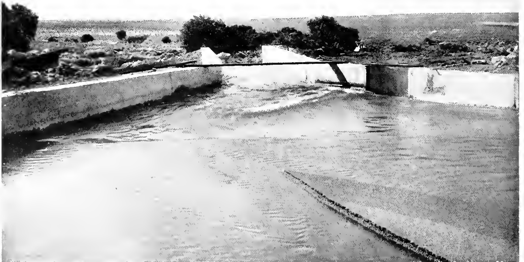
VIAV OF THE MOUNTAIN SECTION WHICH HAS BEEN PIERCED IN THE JAWBONE DIVISION OF THE LOS ANGELES AQUEDUCT SYSTEM,
