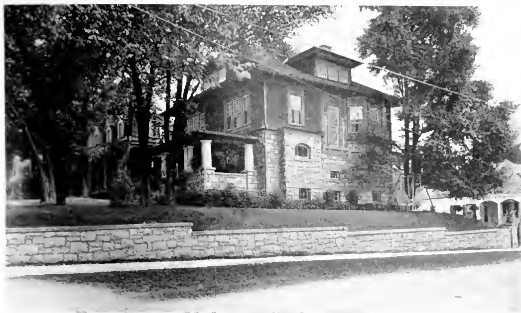
A SIDE VIEW OF MR. STRASSNER'S HOME, SHOWING INTERESTING WALL, IN HARMONY WITH STONE FOUNDATION, AN IMPORTANT CONSIDERATION IN GARDEN-MAKING.
