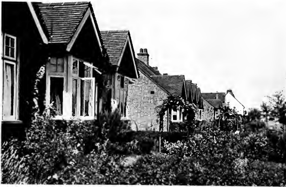
MODERN GARDEN CITY HOUSES THAT HAVE THE CHARM OF ANTIQUE DWELL- INGS, AT PORT SUNLIGHT, ENGLAND.
