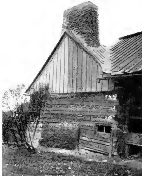
CABIN SHOWING LOOPHOLE WINDOW AND CHIMNEY BUILT INSIDE THE WALLS. IT WAS BUILT IN 1765 AND IS NOW USED AS A REST HOUSE FOR GOLF PLAYERS.
