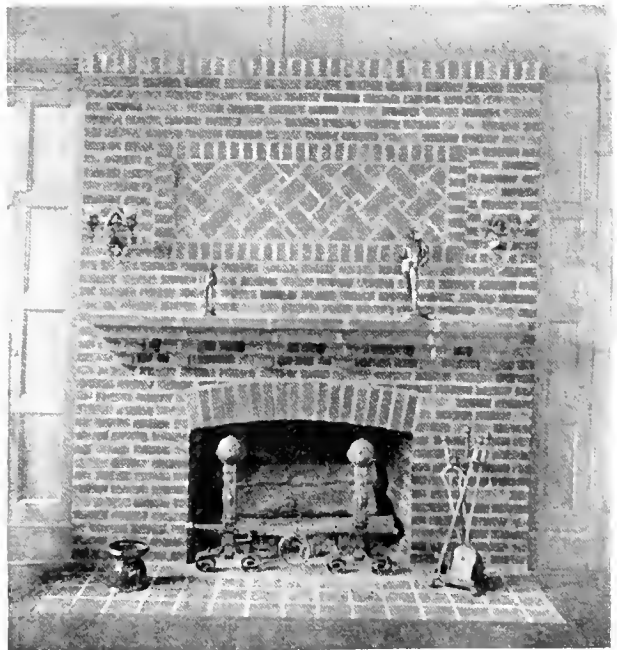
CHIMNEYPICE OF SIMPLE CONSTRUCTION, ATTAINING DECORATIVE CHARM THROUGH THE VARIED TONES OF THE BRICK.
