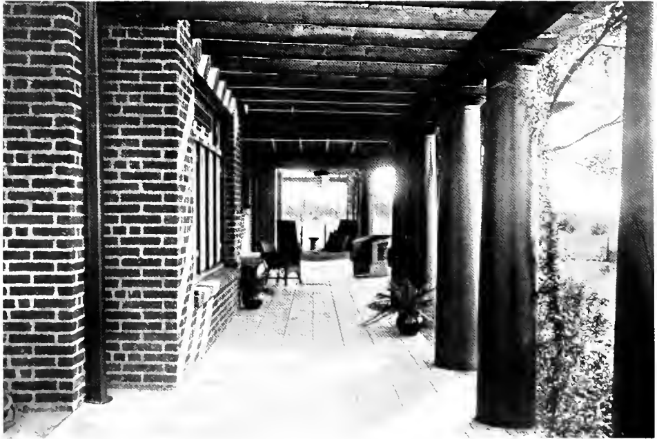
A SIDE VIEW OF "DUMBLANE" WITH GARAGE IN THE REAR. UNDER THE PERGOLA WHICH CIR- CLES THREE SIDES OF THE HOUSE.
