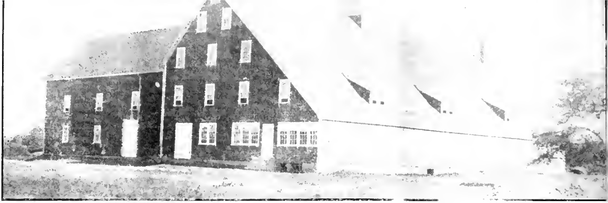
The Big Federal Screenhouse
