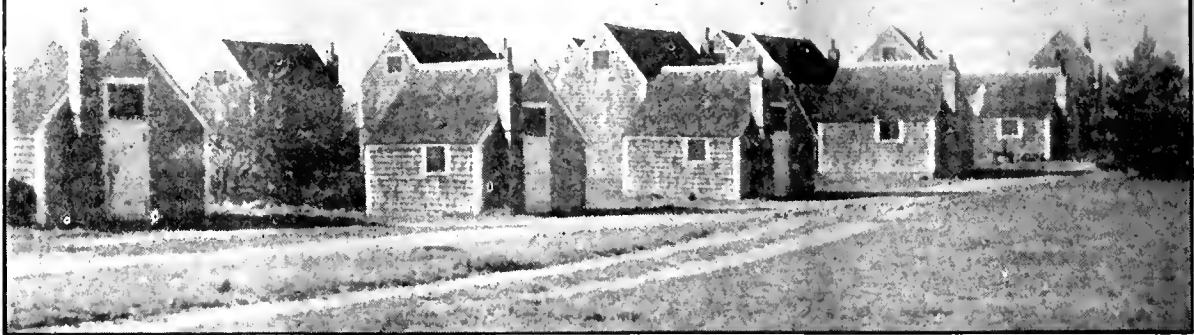
A Section of Federal Village
