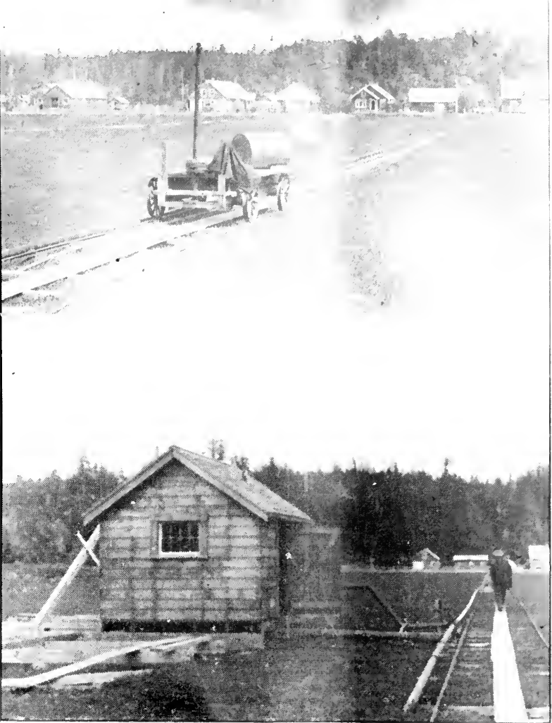
Top—Sprayer rolled out on its tracked-over, boarded-in ditch. Lower—Sump house and sump in the center of a Grayland bog.
