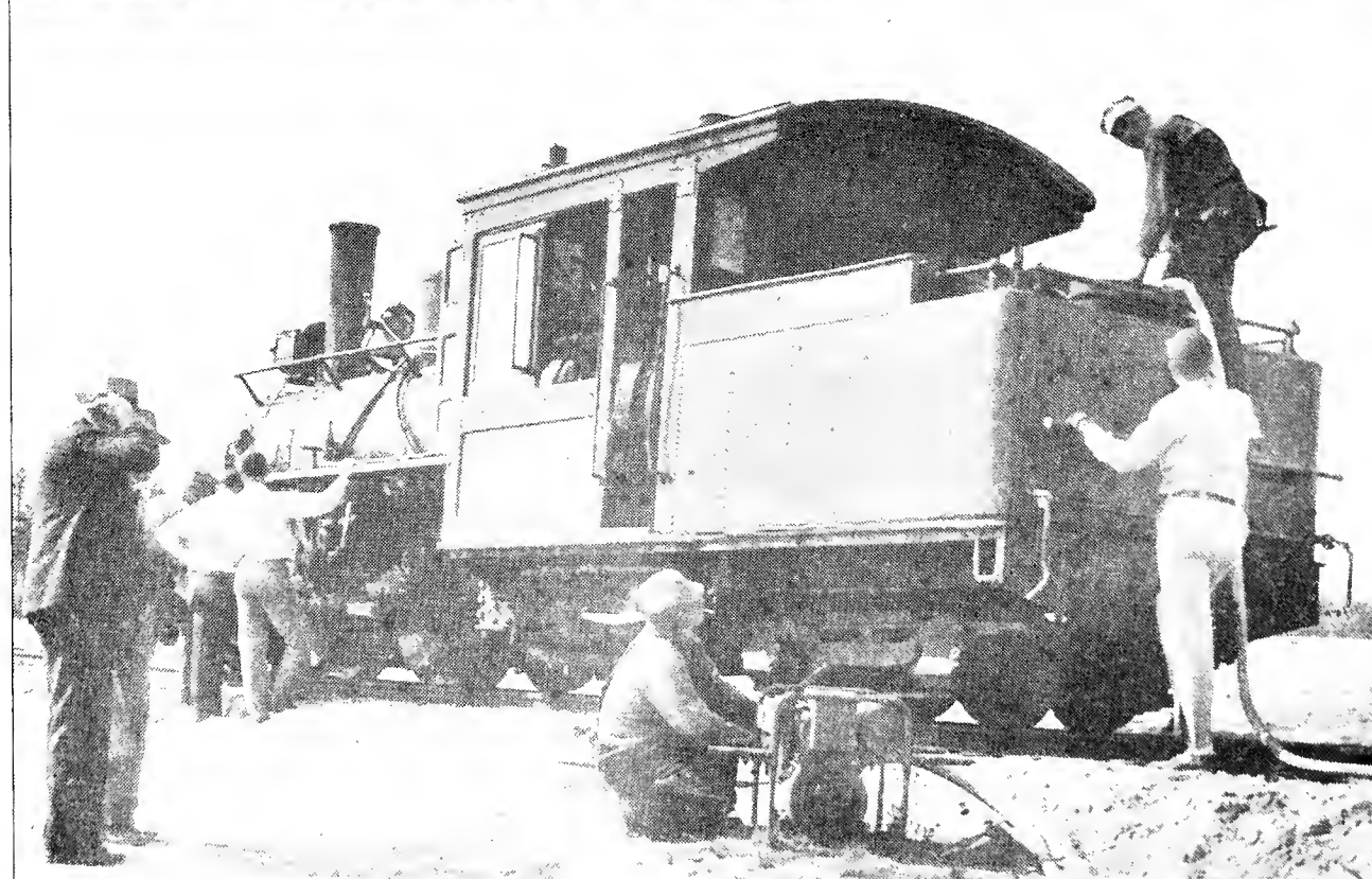
TOP—Crew working at switch. LOWER—No. 7 takes on water at reservoir
