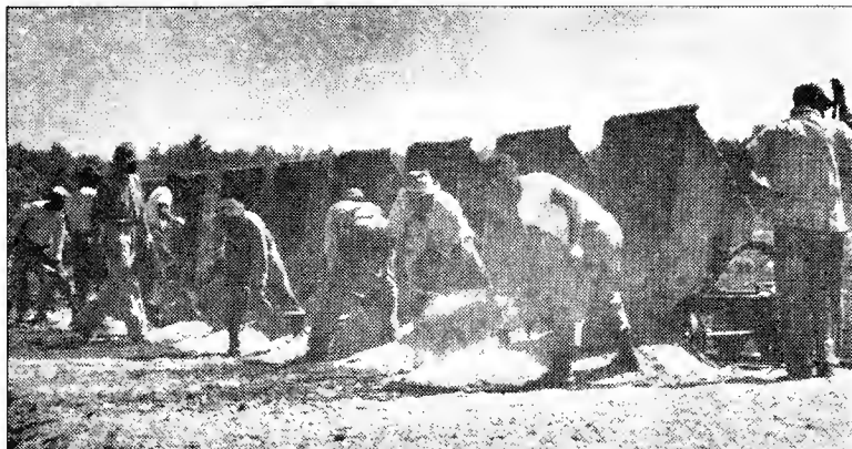
Top—Men spread sand, dumped from cars run out on track over bog. Lower—Shovel dumps sand into the screen, and it pours through into cars as they pass beneath. Scene is in enormous pit of Halifax bog, taken from top of opposite bank.
