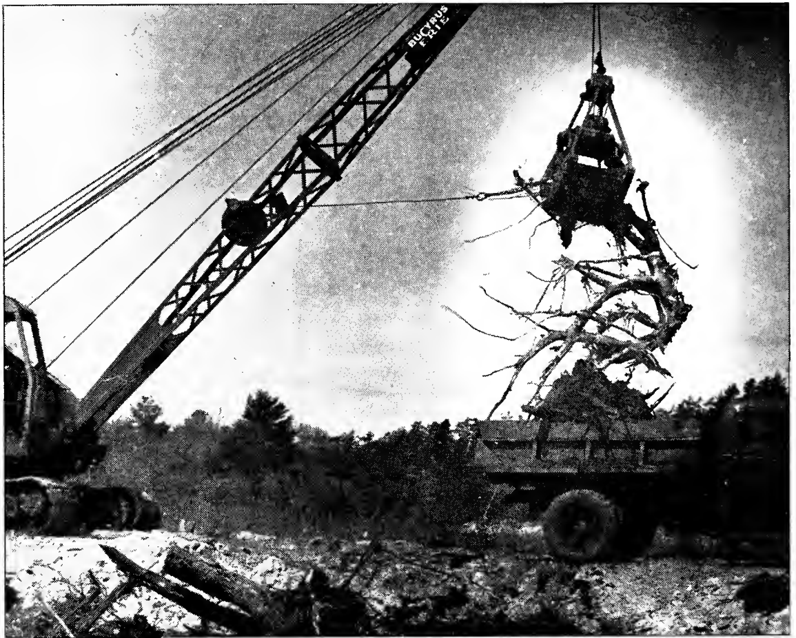
Gault Crane swings big stump from bog to truck standing on dike roadway.
