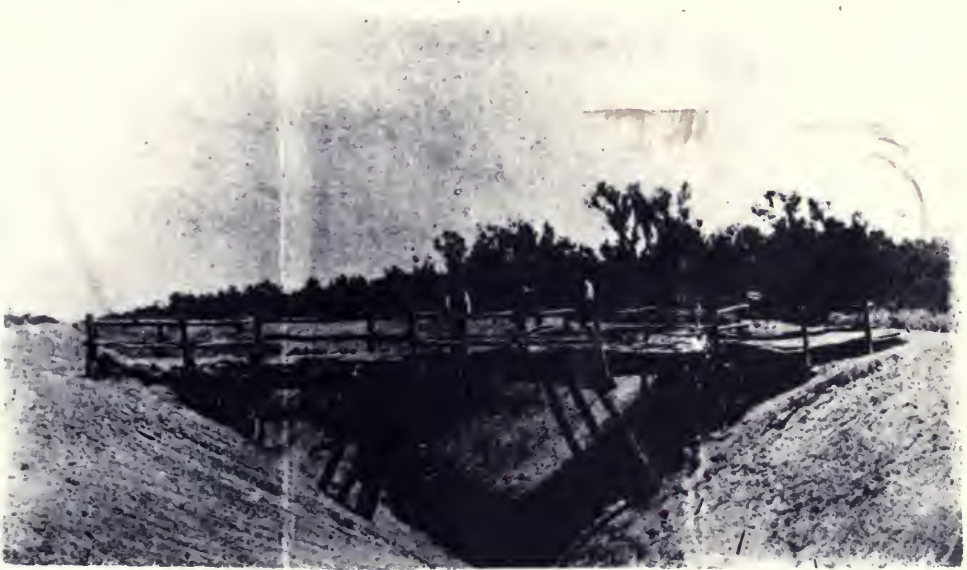
18 — Bridge over Ditch near Catwood, March 10, 1892. The bridge is made of mesquite timber
