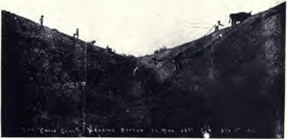
This was the plan of the canal. The ditch had to be dug to a depth of 100 feet. The teams of horses were worked on top and pulled in shafts up the side.
