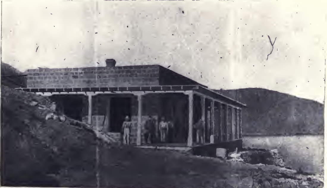
2.—The Custom House is 50 x 40 feet, with a 10 ft. wide porch on three sides. It is built of red porphyry, and is on the southeast corner of the block, 600 x 300 ft., which is reserved for Federal offices. Pioneer Cove is plainly seen to the east. The cost was $8,000 Mexican silver, and was entirely the work of the colonists, who
