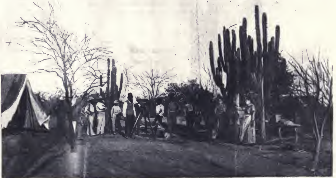
21.—The first dwelling place in Mochis—the tent of Mrs. Herring. Engineer Herring stands close by his transit.
