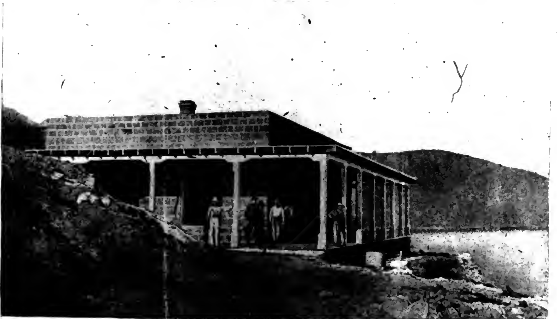
The Custom House is 50 x 40 feet, with a 10 ft. wide porch on three sides. It is built of red porphyry, and is on the southeast corner of the block, 600 x 300 ft., which is reserved for Federal offices. Pioneer Cove is plainly seen to the east. The cost was $8,000 Mexican silver, and was entirely the work of the colonists, who
