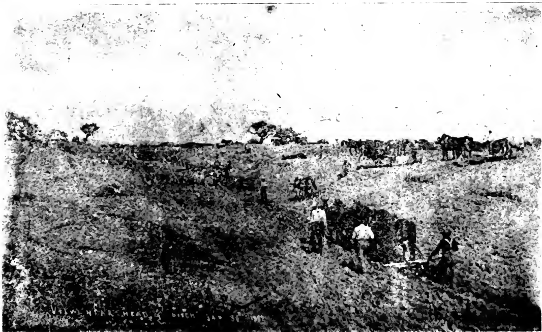
4. After the stumps were removed, by the choppers and grubbers, then the six and eight-horse plows were used. The wheel scrapers with two horses followed and took the earth to the top and dumped it on the sides.
