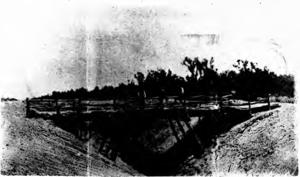
18 — Bridge over Ditch near Catwood, March 11, 1892. The bridge is made of mesquite lumber
