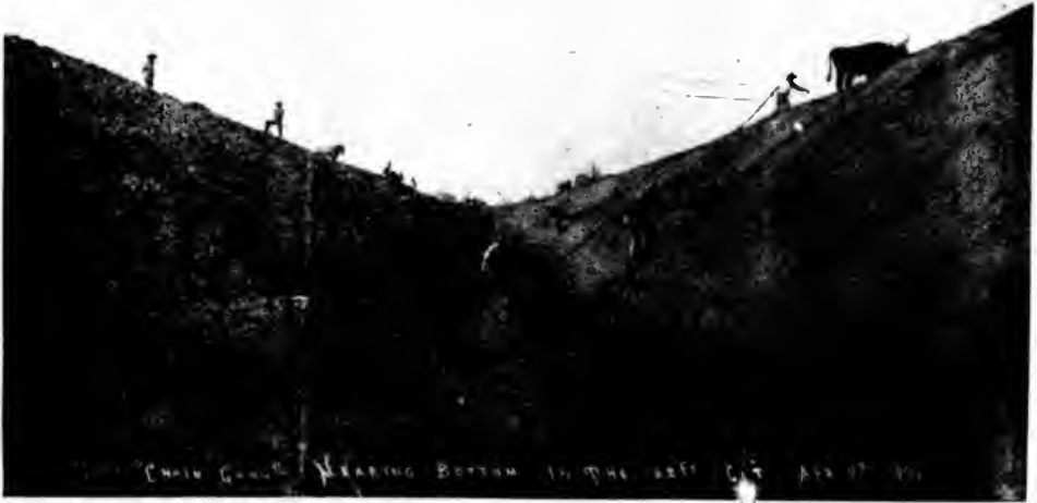
100—The erosion of the gully in the distance is not below ten feet deep. The teams of mules are worked on top and pulled in shovels up at the side.
