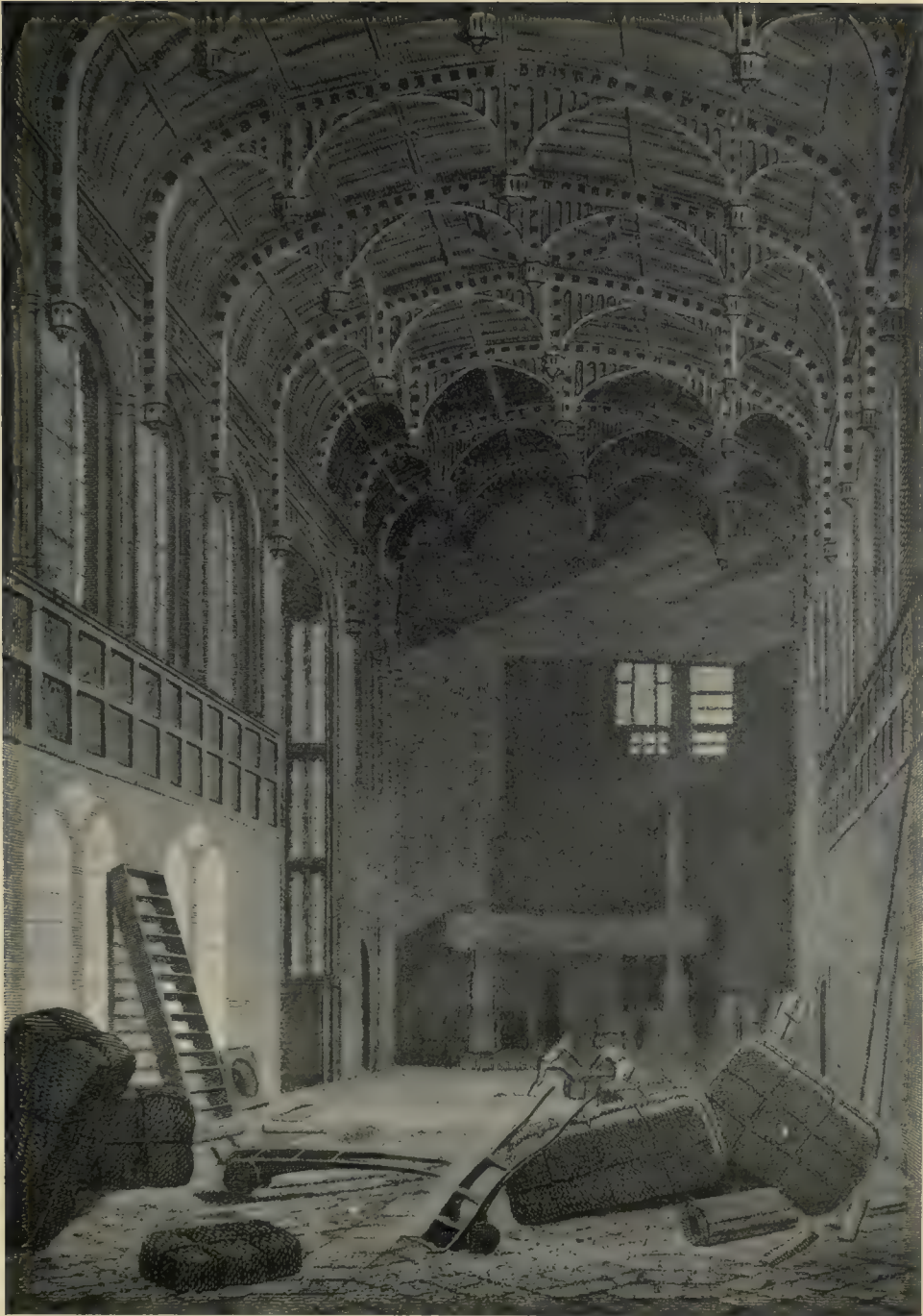
GREAT HALL LOOKING NORTH, 1804
