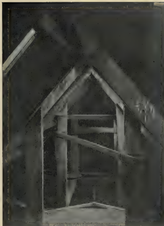
TIMBERS IN ROOF OF HALL
