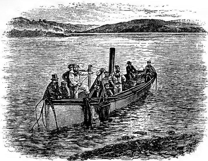
DREDGING ON THE PARAMATTA RIVER, SYDNEY.
