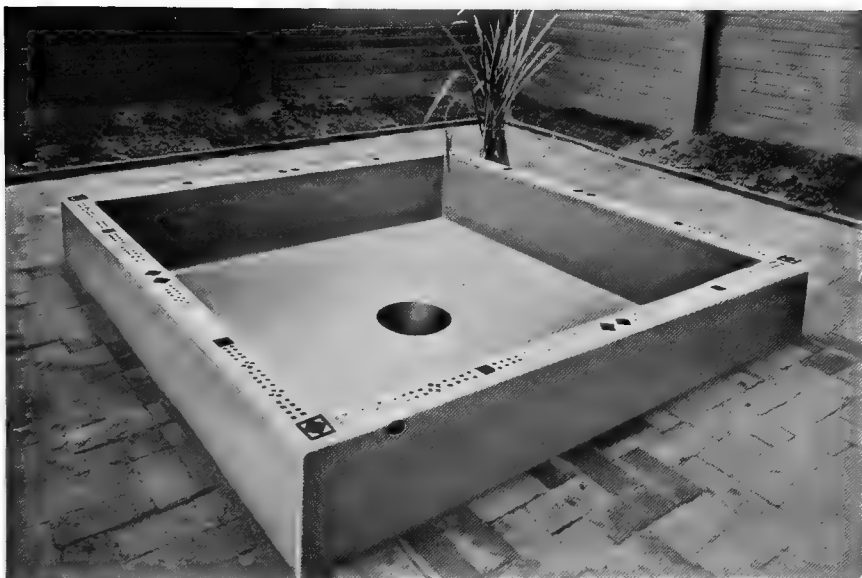
FIG. 167. FINISHED POOL, SHOWING SUNKEN LILY POT AND OVERFLOW
