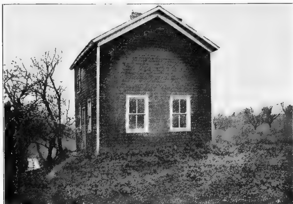
Fig. 71—Shop (looking South).
