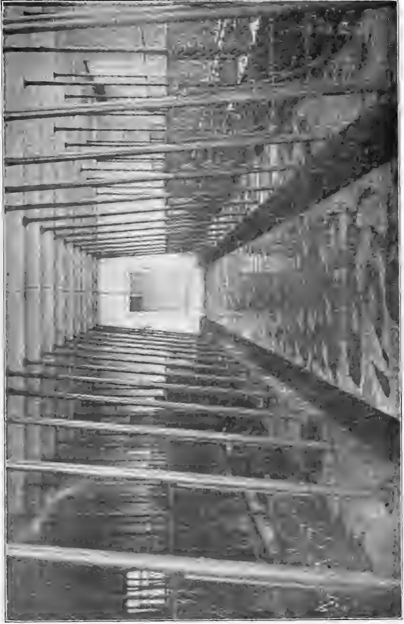
Fig. 99.—A sanitary dairy barn. Cement floor, iron stalls, sides whitewashed, well lighted, and provided with a good system of ventilation. Exterior shown in Fig. 100. (Report of Kansas State Board of Agriculture, No. 87, 1903.)
