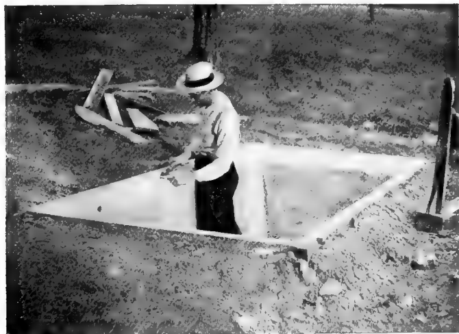
The tank is 8 x 4 ft. and was made of concrete. It cost $11.28 all told (For details see page 29)
