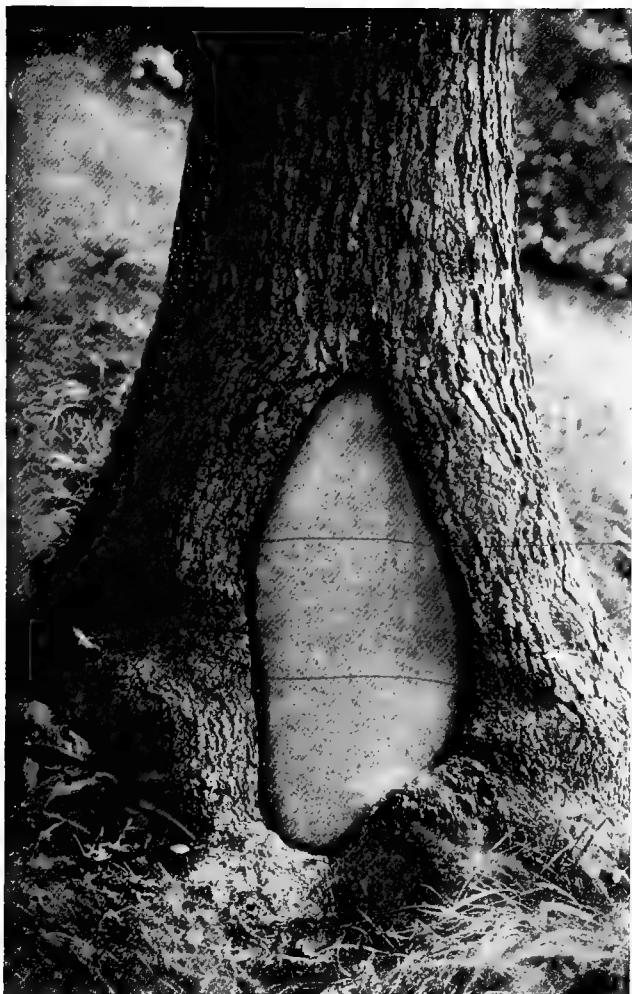
Cavity in the base of a white oak filled with concrete
