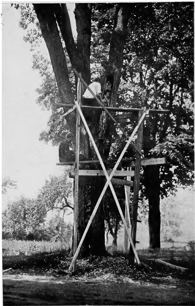
Excavating a large cavity
