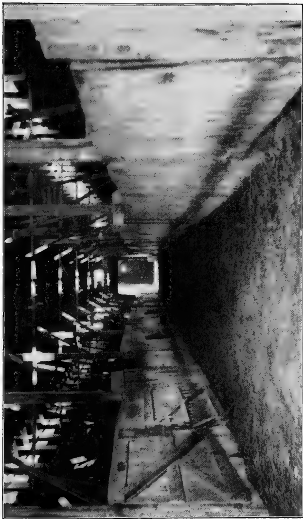
INTERIOR OF ONE OF THE LARGE BARNs AT A SHEEP-FEEDING STATION ADJACENT TO CHICAGO. Each pen, as shown on either side of the central alleyway, holds about one carload of sheep, allowing six square feet per animal. Note the open windows, which provide ventilation, — an essential to a good sheep barn.
