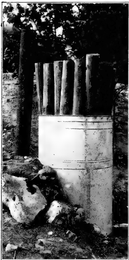
FIG. 55. — Single tank for treating posts.
