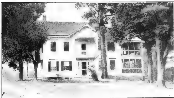
FARMHOUSE WITH OUTSIDE SLEEPING ROOMS
