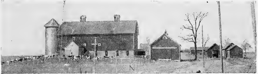
This barn is well located, the yard sloping from the building on all sides.
