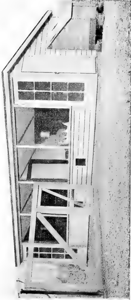
An ideal home poultry plant designed at the Purdue University Experiment Station. The glass window extends almost to the floor and there are muslin curtains for the openings
