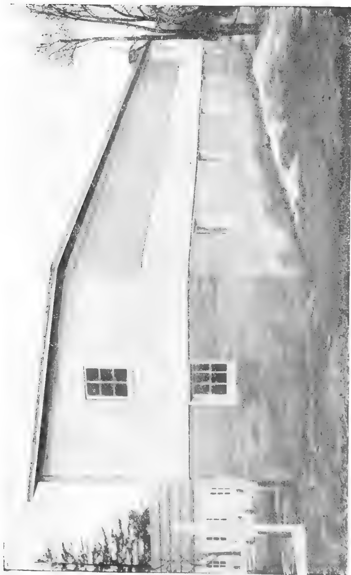
Incubator building. The lower part of the above unit is the incubator cellar, which has a capacity of 40,000 chicks per season. It is a hot water system. The upper part is used for a laying house. The building is 14x30 feet.
