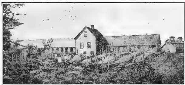
FIG. 14—HOUSE AND YARDS AT NEW YORK EXPERIMENT STATION
