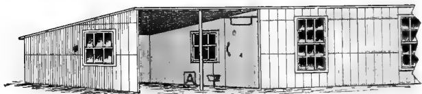
FIG. 2—THE ORIGINAL SCRATCHING SHED HOUSE
