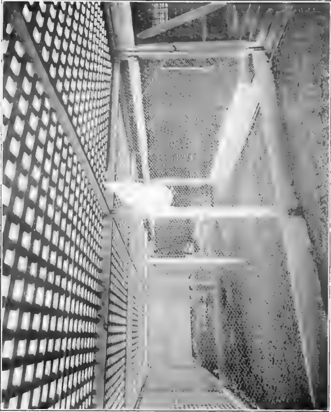
Inside view of lattice yard of brooder house.
