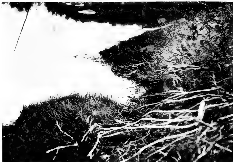
A gate or spillway cut in the dam in order to let the surplus water escape. In times of drought this would be either partly or completely closed.
