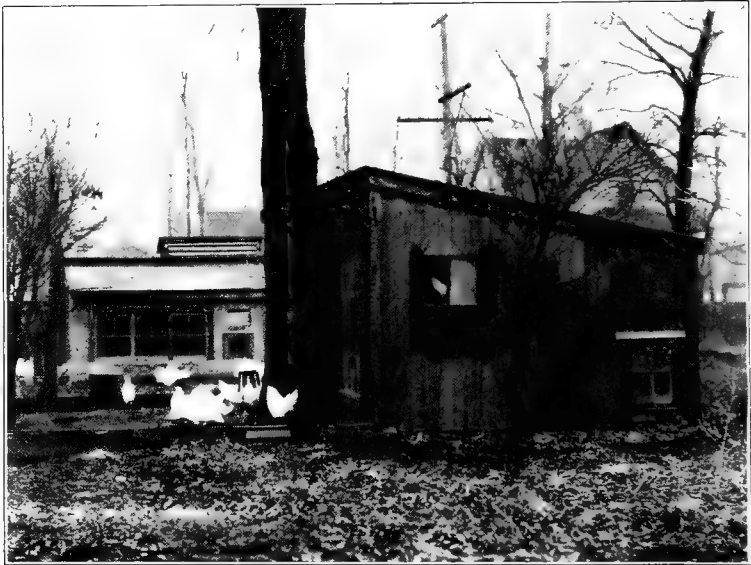
View Showing the Two Houses Used in These Experiments
