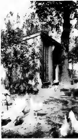
End View of Pullet House
