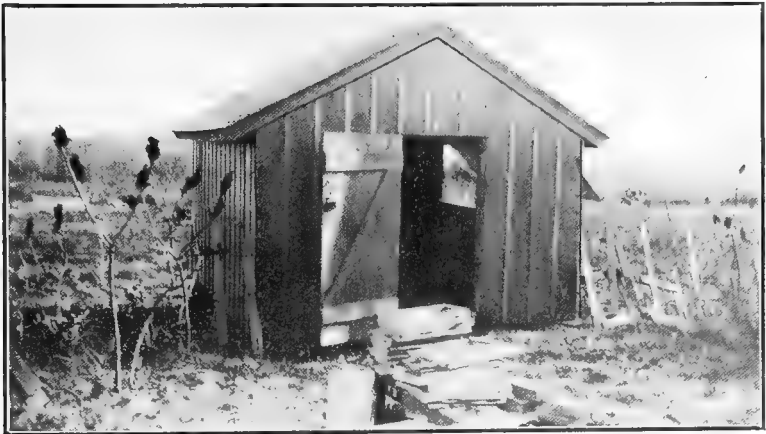
FIG. 24.—Extracting House at Hammond Hill, R I., 1916. Screened openings on each side give ample ventilation.
