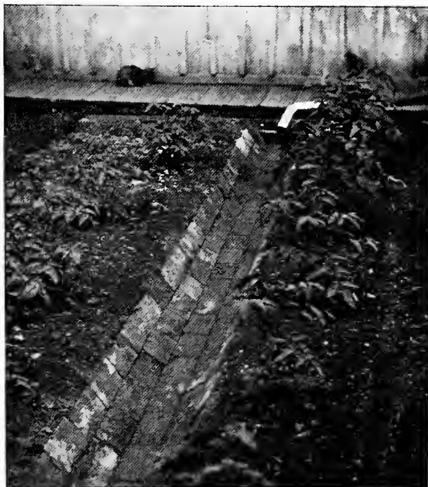
Fig. 10.—Surface-drain Made of Ordinary Bricks, Showing Delivery-pipe from Kitchen Sink and Bath.
