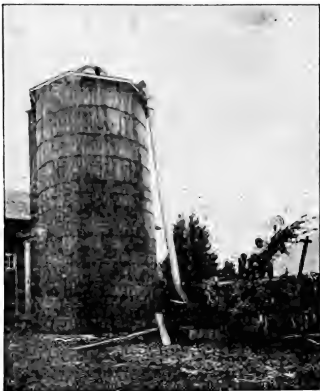
Fig 43—Filling Silo with Blower
