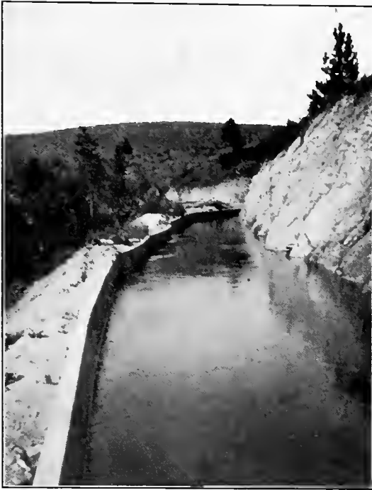
FIG. A.—Side hill canal with retaining wall used to replace wood bench flume, Hedge canal, Montana.
