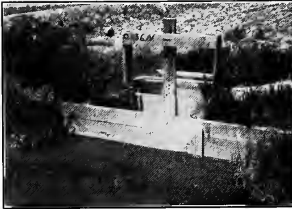
FIG. C.—Headgate with sharp edged orifice set in front wall, Minidoka project.
