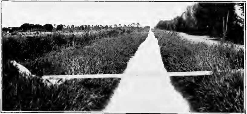
FIG. D.—Similar canal to that shown in Fig. C. with excessive growth of vegetation, value of n = 0.029 (Figs. C and D from Bull. 194, U. S. Dept. of Agric.)
