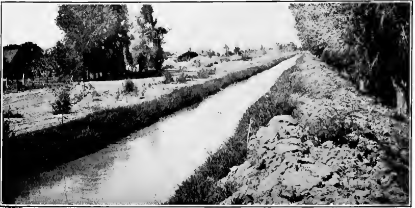
FIG. C.—Canal in Imperial Valley shortly after cleaning, value of n = 0.022 .
