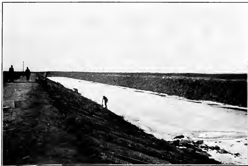
FIG. B.—Main canal Minidoka project, lined with sage brush preparatory to silting.
