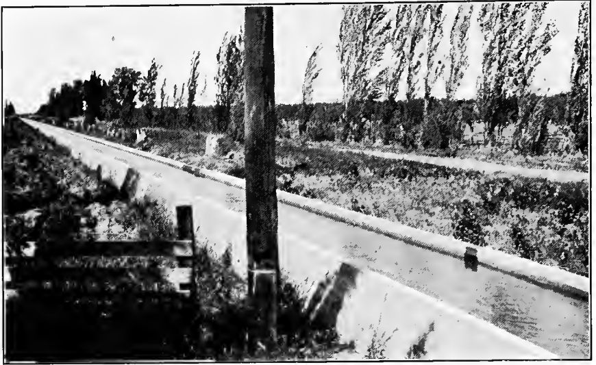
FIG. C.—Concrete flume in light fill in sandy soil, Crocker-Huffman Land and Water Co. California.
