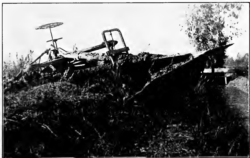
FIG. B.—Canal "V" used to remove silt, Imperial Valley.
