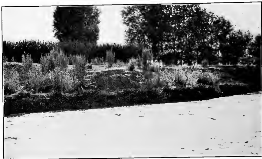
FIG. C.—Brush riprap used in the Imperial Valley.
