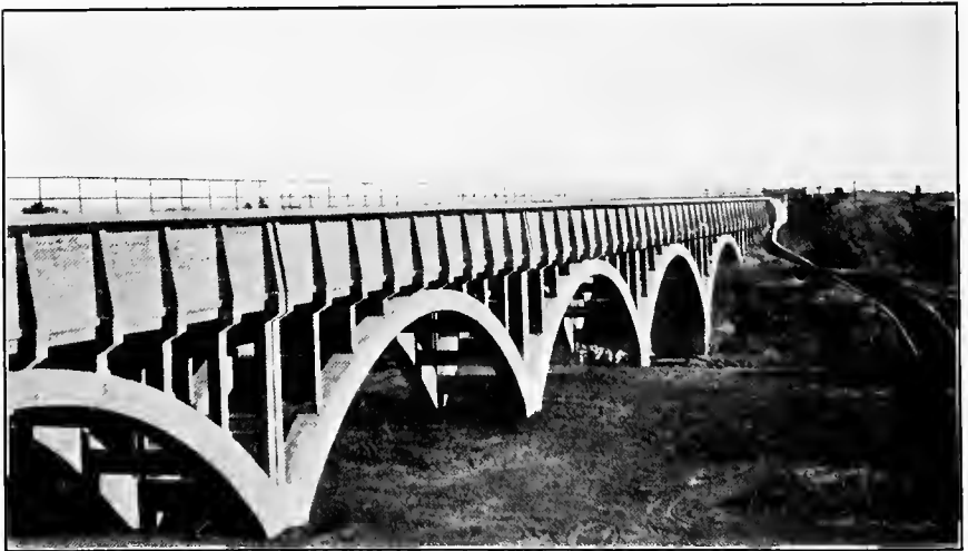
FIG. D.—Concrete arch flume used to replace wood flume, Modesto irrigation district.
