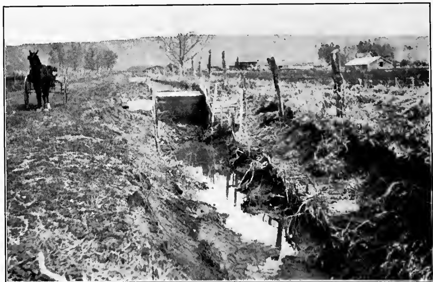
FIG. D.—Willows used to reduce erosion, Snow Lateral, Billings, Mont.
