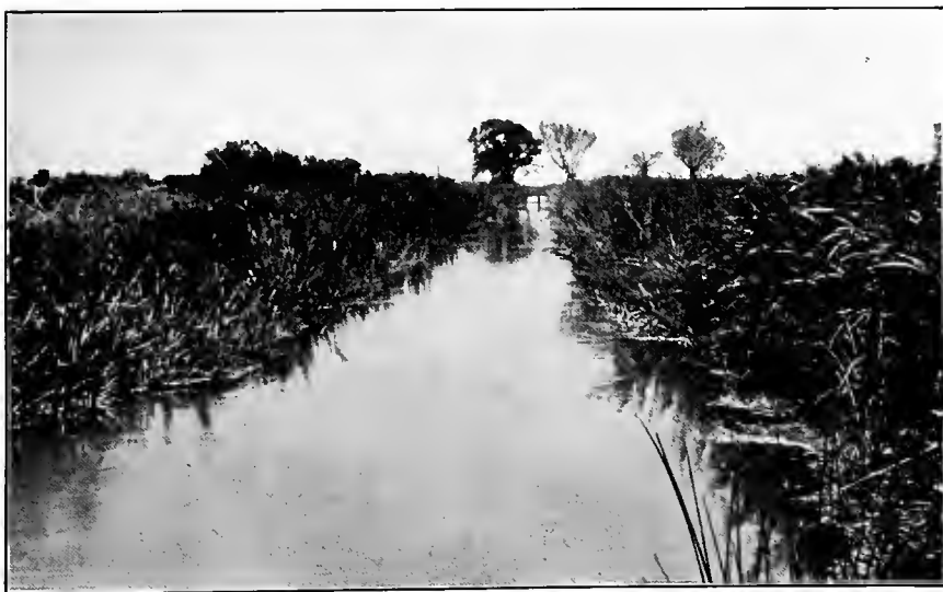
FIG. B.—Vegetation at sides of canal, causing silt berms.
