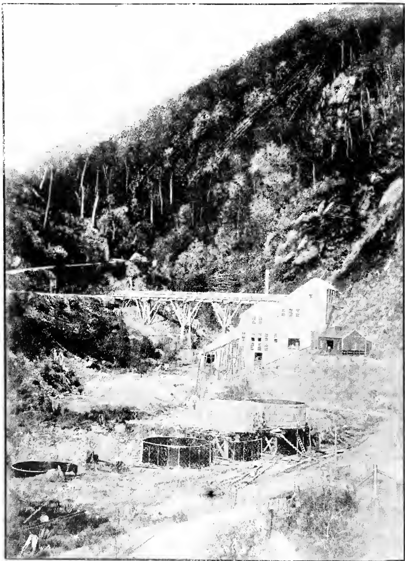
GOLDEN FLEECE MINE, REEFTON: GENERAL VIEW OF BATTERY, BRIDGE, CYANIDE TANKS, ETC.
