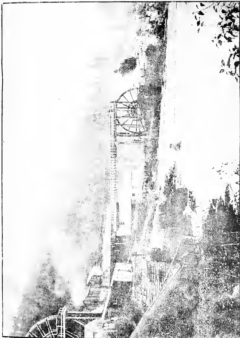
WEALTH OF NATIONS MINE, REEFTON, SHOWING PORTION OF OLD 50 FT. DIAMETER OVERSHOT
