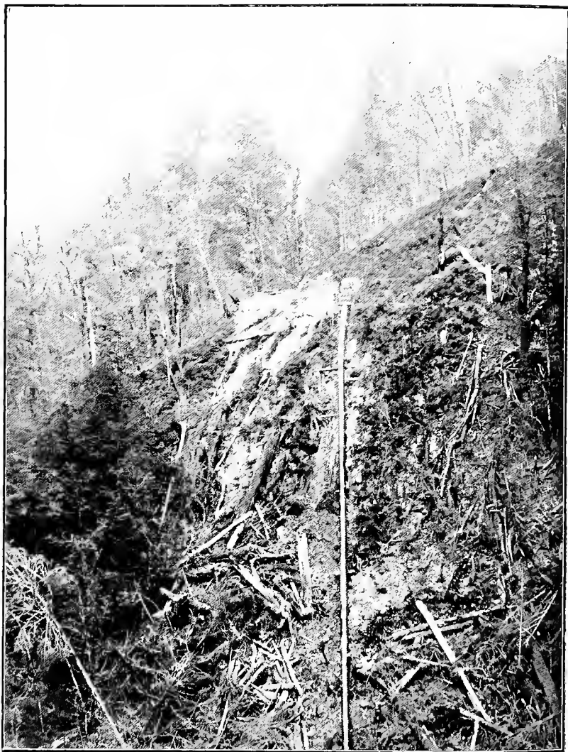
PROGRESS MINES OF NEW ZEALAND, REEFTON: SIPHON OF WATER-RACE AT HUT CREEK. Mining Handbook.
