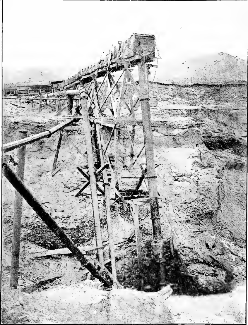
IN ELEVATOR OF CHAMPION HYDRAULIC COMPANY'S CLAIM, BEAUMONT, OTAGO Mining Handbook.
