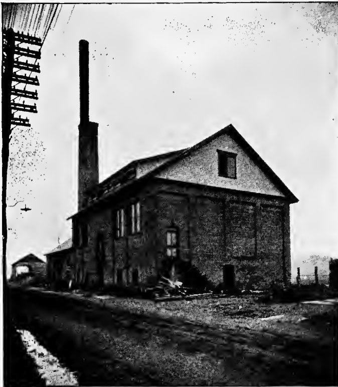
LEHIGH-NORTHAMPTON POWER HOUSE.
