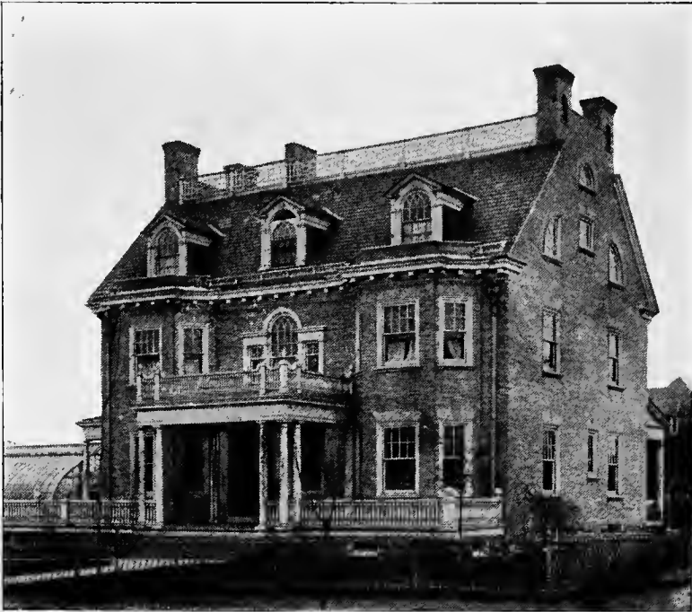
RESIDENCE OF D. G. DERY.
