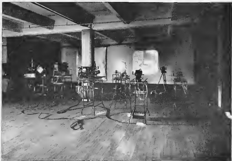
View of Projection Room in use as Dark Room
