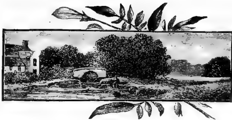
BARCOMBE MILL, RIVER OUSE
