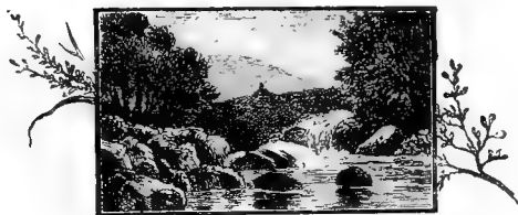
IVY BRIDGE, RIVER ERME, DEVON
