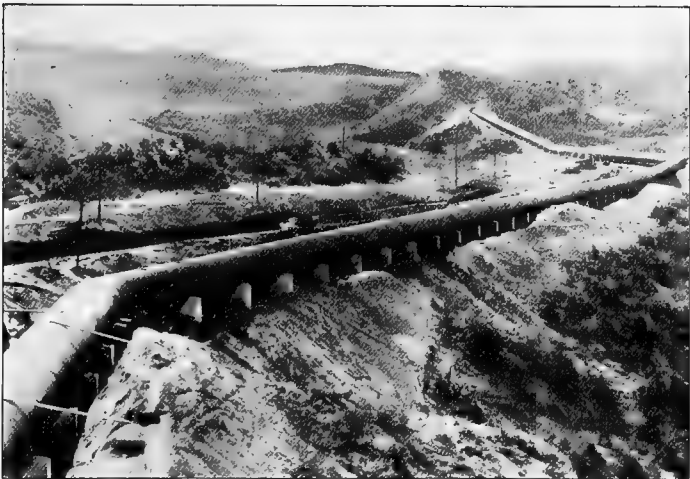
The Owens River aqueduct, through which water is carried to Los Angeles from a source more than two hundred miles distant.
