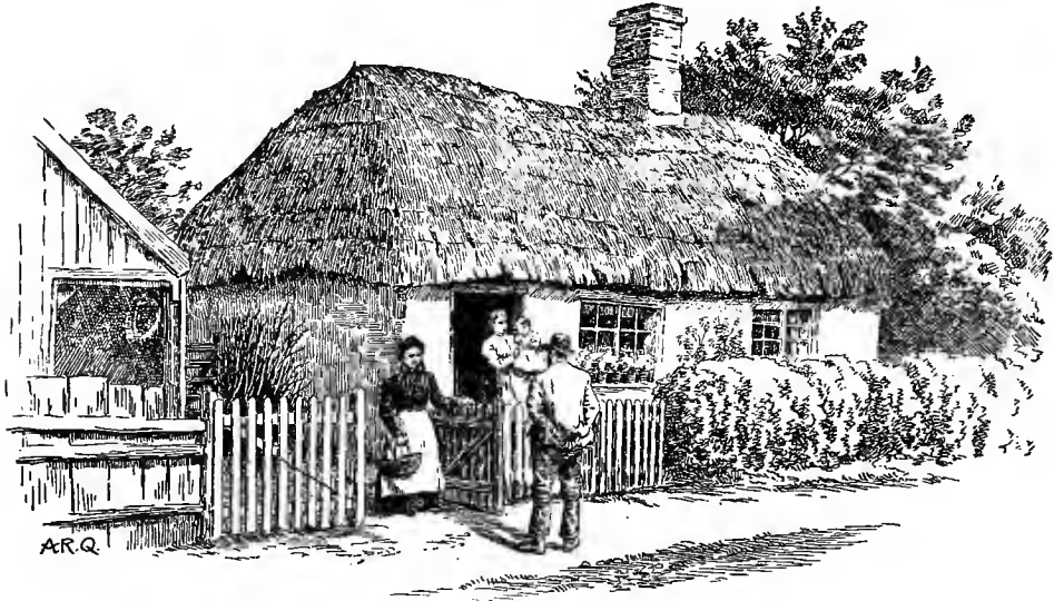
COTTAGE AT ROUTH, YORKSHIRE
