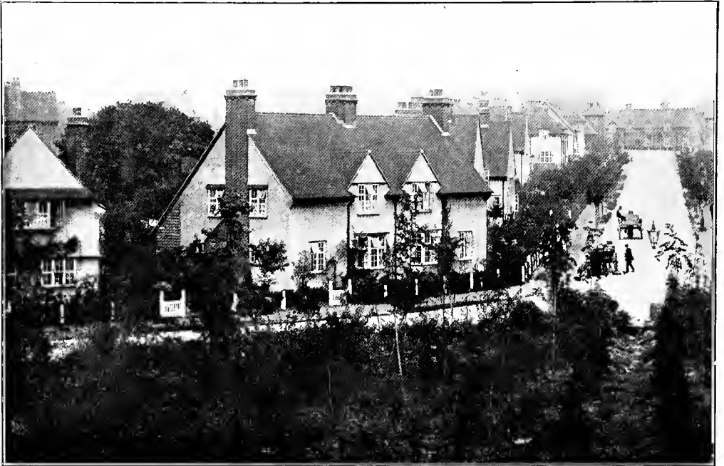
FRONT VIEW AT HAMPSTEAD GARDEN SUBURB, ILLUSTRATING 12 HOUSES TO THE ACRE NET OR ABOUT 10 GROSS.
