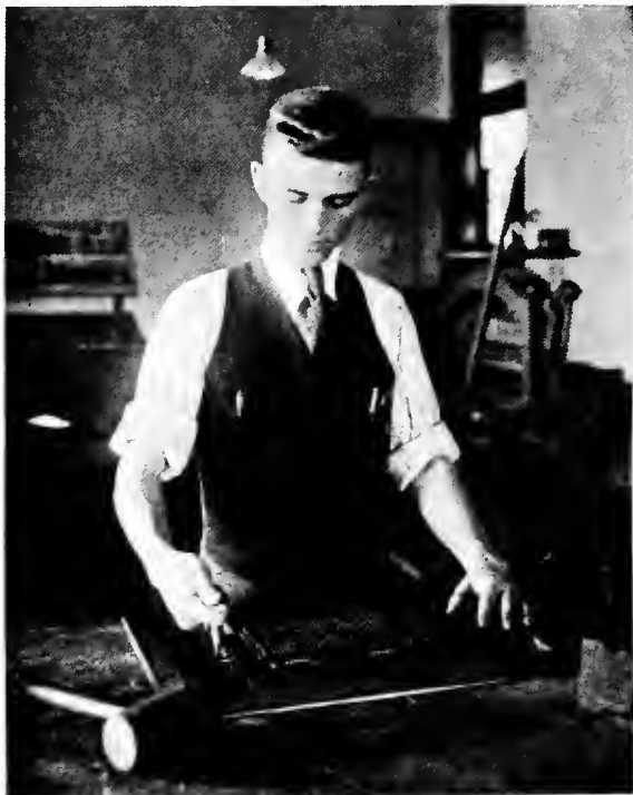
Fig. 58.—Locking of Form in Chase.
