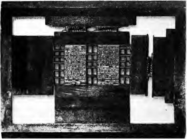
Fig. 61.—Imposition of Two Forms in Chase.
