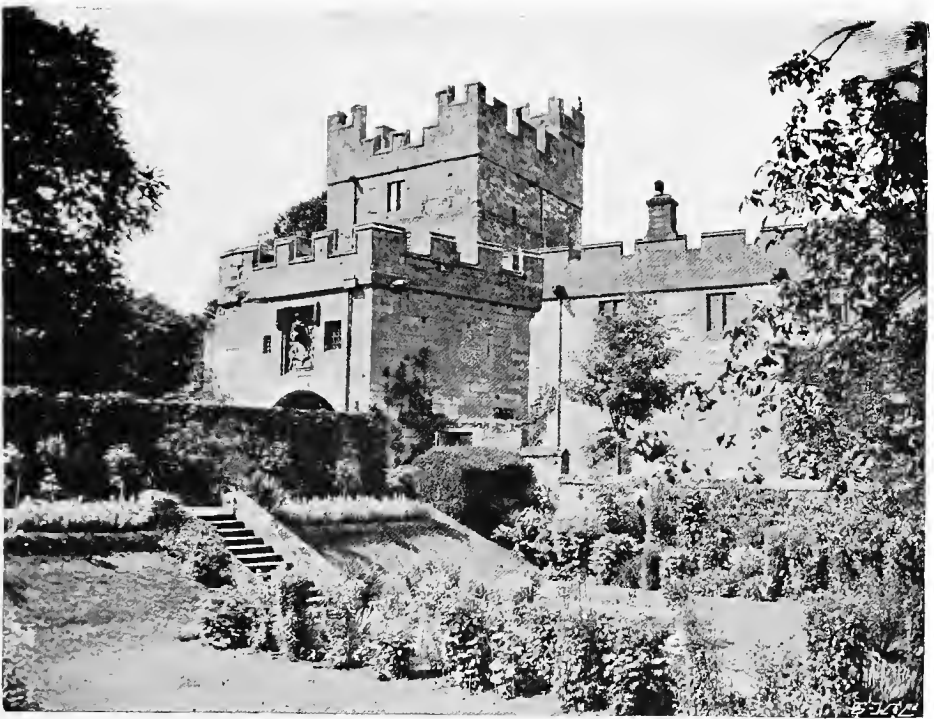
GATEWAY AND DACRE TOWER FROM THE GARDEN
