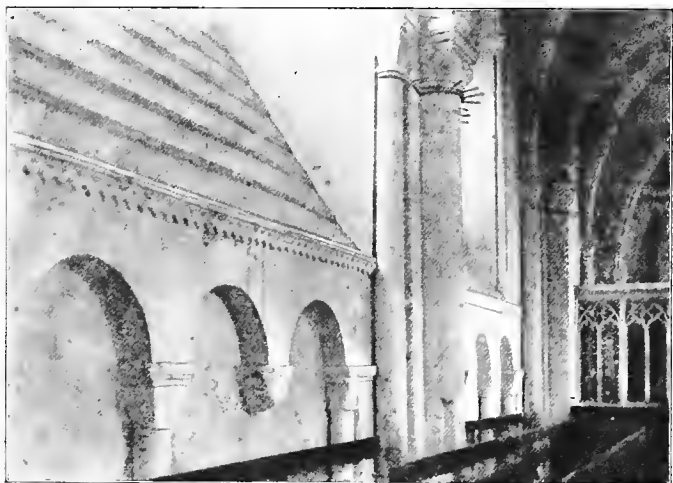
WALL ARCADE, NORTH SIDE,
