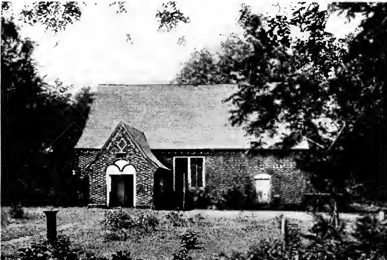
YEOCOMICO CHURCH, WESTMORELAND COUNTY
