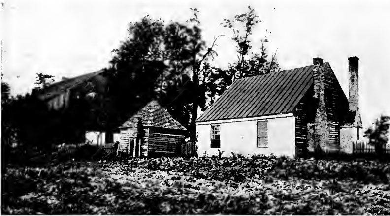
HOUSE WHERE STONEWALL JACKSON DIED, FAIRFIELD, CAROLINE COUNTY
