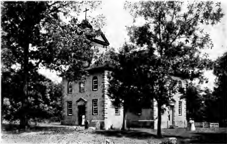
ACQUIA CHURCH, STAFFORD COUNTY
