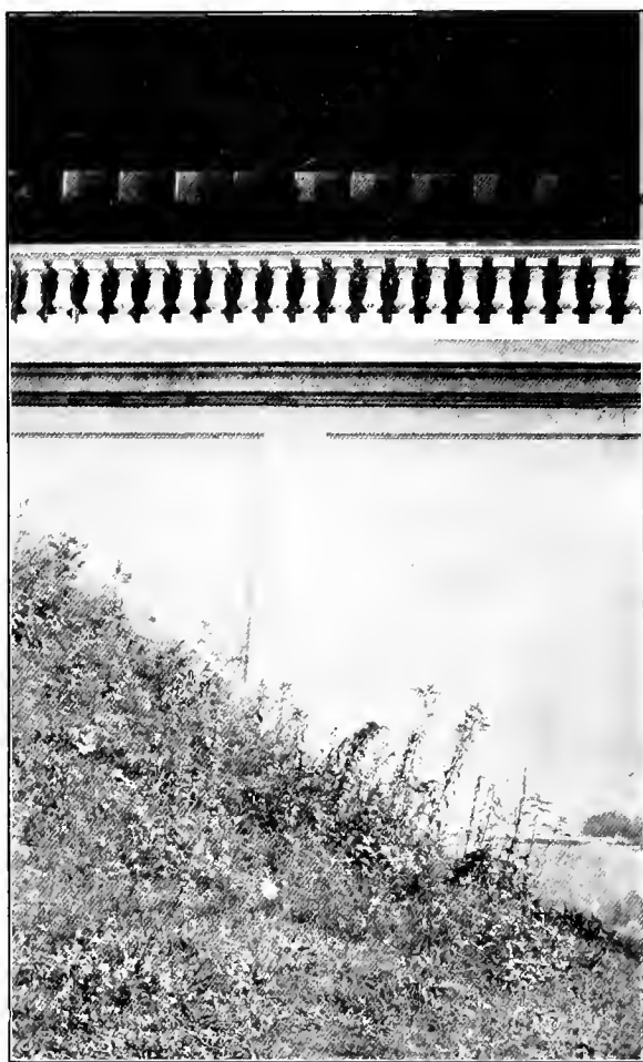
FIG. A.—Ornamental concrete handrail approach to concrete arch.
