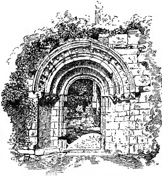
DOORWAY TO CLOISTER. Point 4 on Plan.
