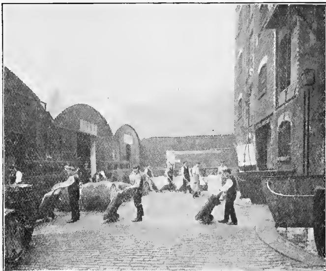
LANDING RUBBER AT NEW CRANE WHARF.
