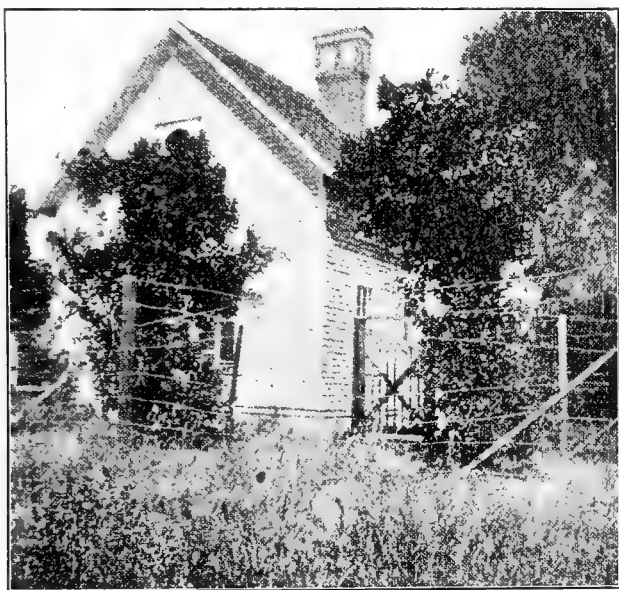
Original Washington Navel orange trees, at the Tibbets homestead, Riverside, Cal. [Removed April 25, 1902, to the head of Magnolia Avenue.]
