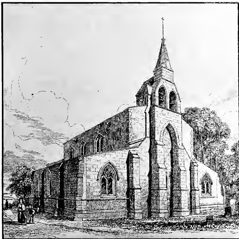
Bell-turret supported on buttresses (Burton Lazars, Leicestershire)
