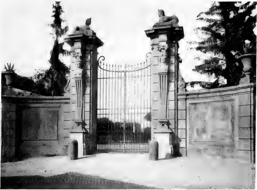
ENTRANCE GATE OF THE VILLA ALBANI
