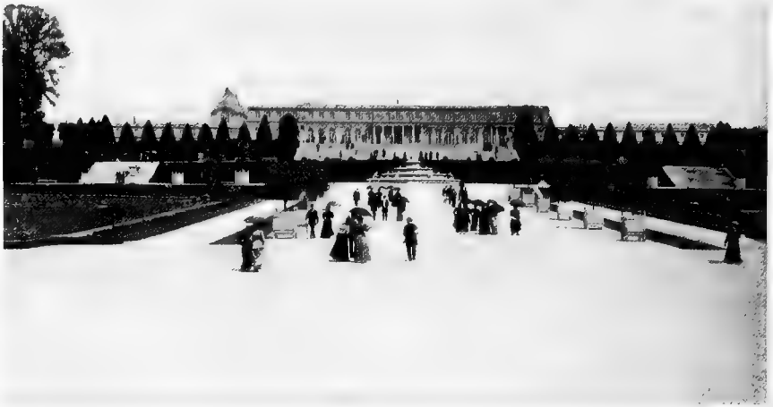
BASIN OF LATONE AND THE PALACE
