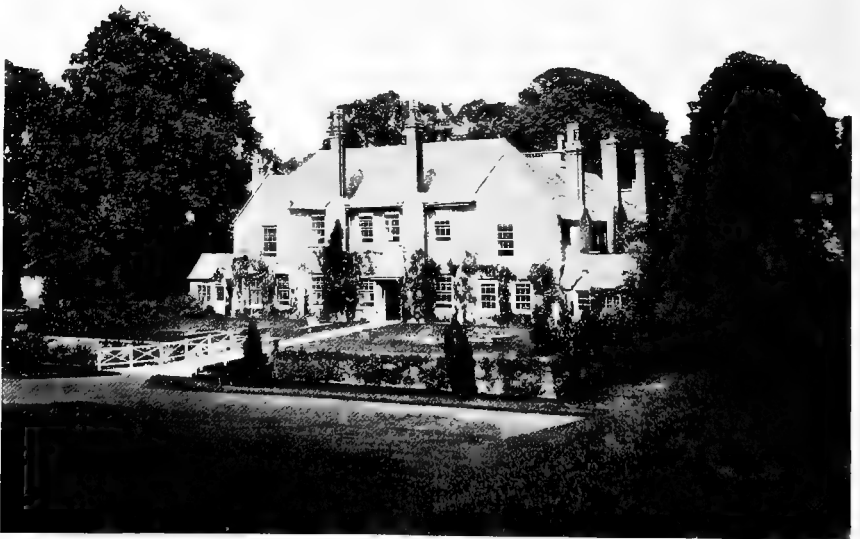
A SMALL HOUSE-COURT
