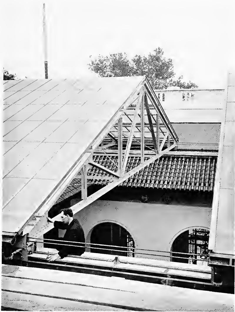
Sliding Roof, Operated by Electricity, Partially Opened Over Patio
