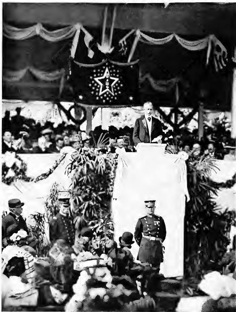
Secretary Root Delivering Address at Corner-stone Laying
