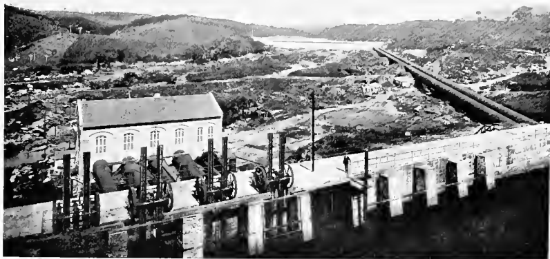
Great Power and Lighting Plant, San Paulo, Brazil
