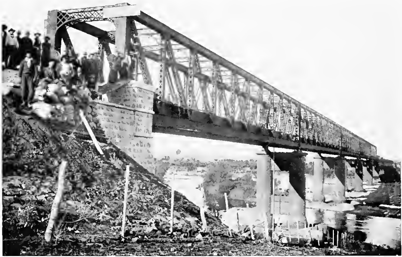
Steel Bridge on One of the Principal Railways of Chile
