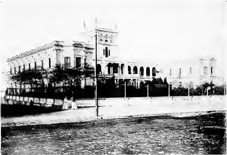
National Building, Asuncion, Paraguay
