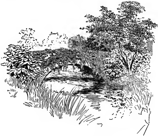
STONE BRIDGE OVER SMALL STREAM
