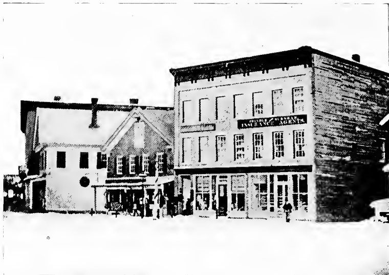
From left to right: Verder's Bakery; Landon & Bates, Hardware; M. Balch, Millinery; Hilliards & Oaks, Dry Goods. Built in 1864. Destroyed by fire 1867. Merchants Row. Located on the present site of Wilson Clothing Co. and Hulett Block.
