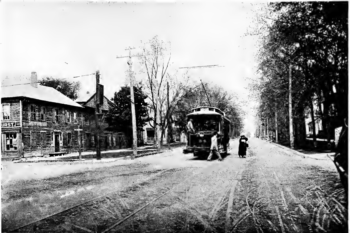
MAIN STREET LOOKING NORTH FROM WEST STREET.
