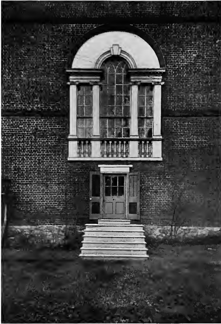
PALLADIAN WINDOW IN CHASE HOUSE
