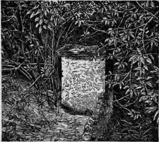
CHIMNEY OF A HOUSE BURIED IN SAND.
